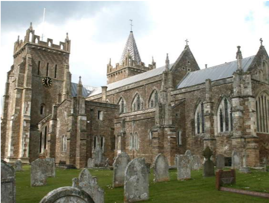
Fig 41: The Church of Ottery St Mary, viewed from the southeast
