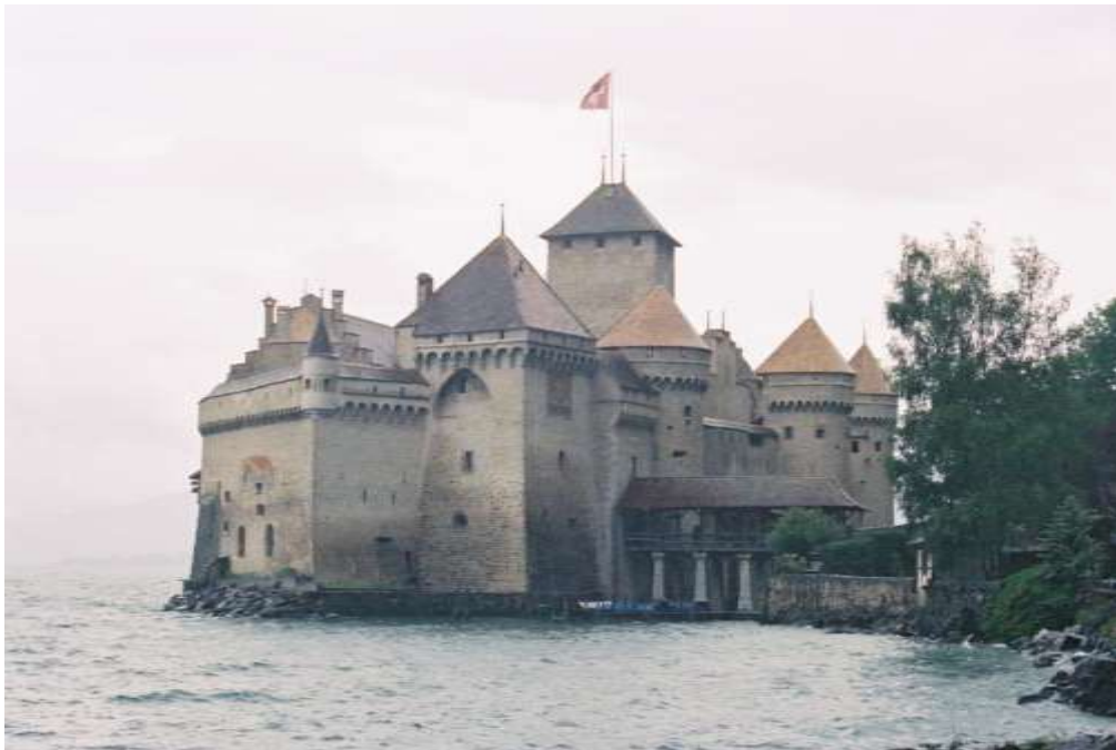
Fig 13: Chillon Castle, Switzerland
