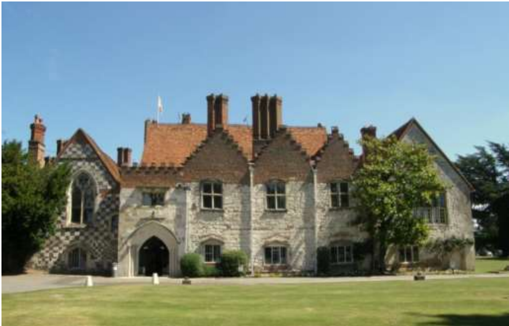
Fig 18a: Bisham Abbey south front showing, on the right of the building, the remaining front of the 14 th century cloister added to the Knights Templars’ preceptory at Bisham by William Montacute, 1 st Earl of Salisbury. The front between the Templars’ entrance porch and Salisbury’s cloister was added on to the Templars’ Hall in the 16 th century
