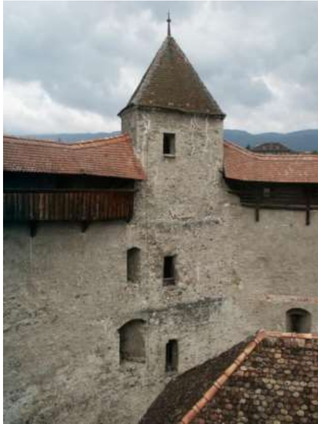
Fig 26d: A “D”-shaped Tower of the Petit Chateau with a shouldered arch at first floor level
